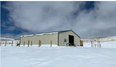
A new barn at the MW Ranch will be the new home for Education Horses, making room once again for the Unwanted herd at the Farm
