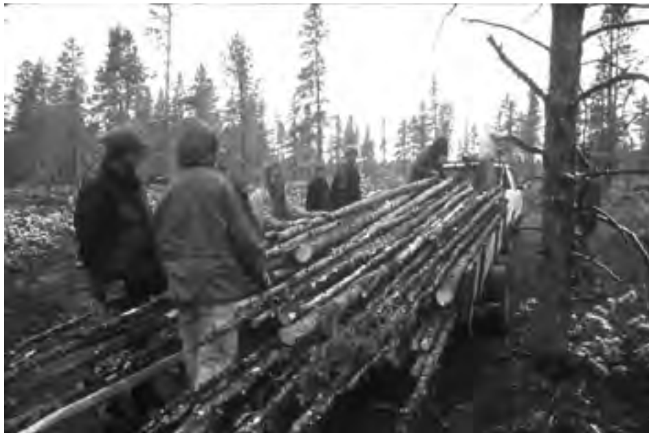
Mission:Wolf staff members A'Lissa, Josh, Kent, Tamas, Thomas and Traci, along with Lenka, George and Sam from SCI load logs onto the trailer while gathering tipi poles and hand rails near Leadville, CO.
